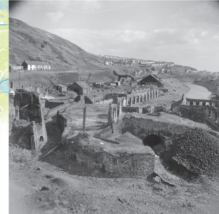
**3.** The exterior west wall of one of the buildings nearer to the river and just to the north of the excavated river dock. Note also the brick archway which appears to have been given a ‘first floor’ connection to the adjacent building.
