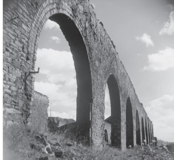
**8.** Westward wall of the ‘Great Workhouse’. This was one of the first buildings on the site, designated to hold over 20 copper reverberatory furnaces. It was the first such building to adopt a long and narrow format with the furnaces arranged primarily so that their grates were near the arches (good air supply) and their chimney flues central permitting better support from the high roof.
