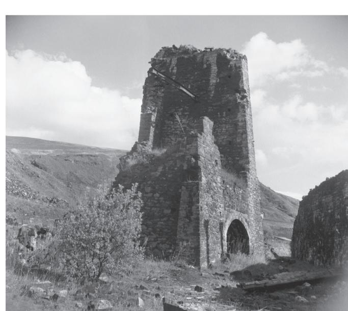
**10.** The incline support tower with its enigmatic archway in the base. The archway forms what appears to be either a hearth or flue exit. It has been suggested that it was once a blast furnace or a lime kiln. However, it was built at the time of the incline itself and how it could have functioned as such is very much open to conjecture given its location relative to other adjacent structures.
