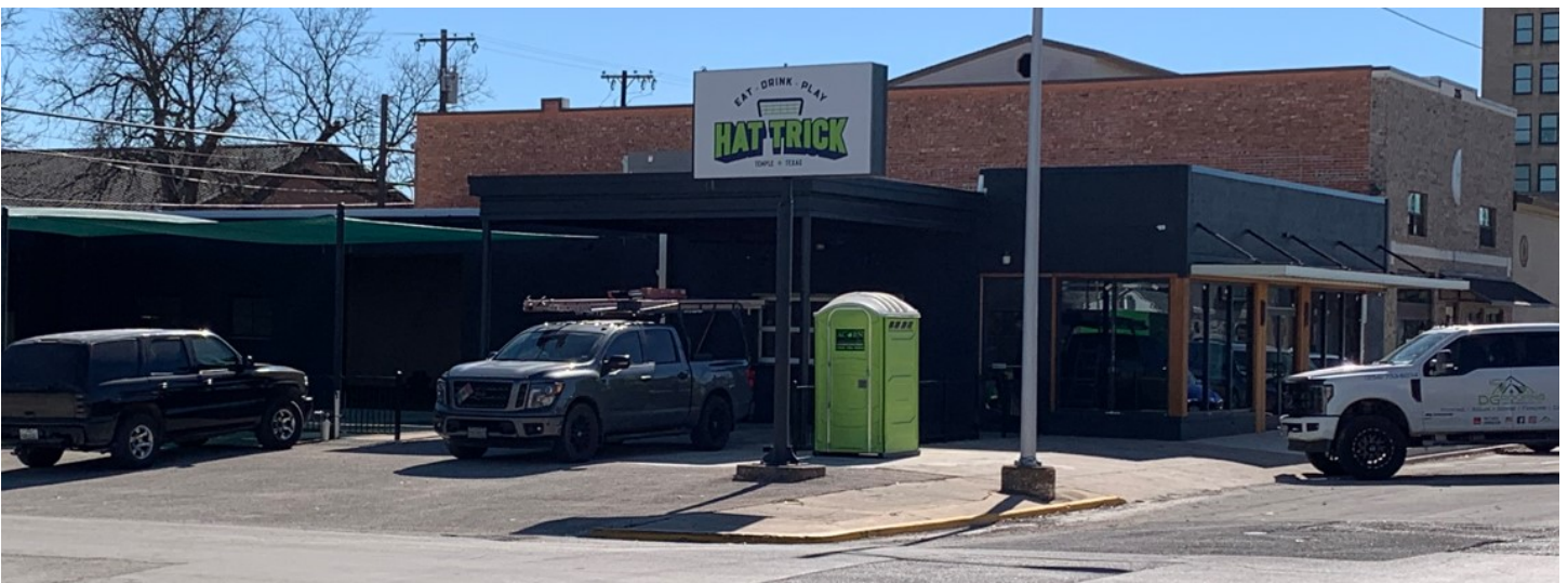
Work on Hat Trick Sports Bar at 217 N Main Street is nearly complete
