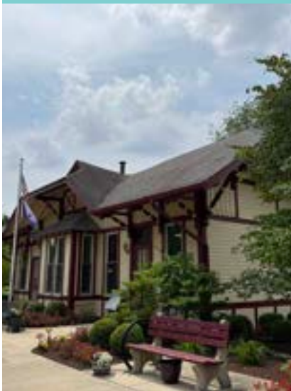
Parke County Visitor's Center
