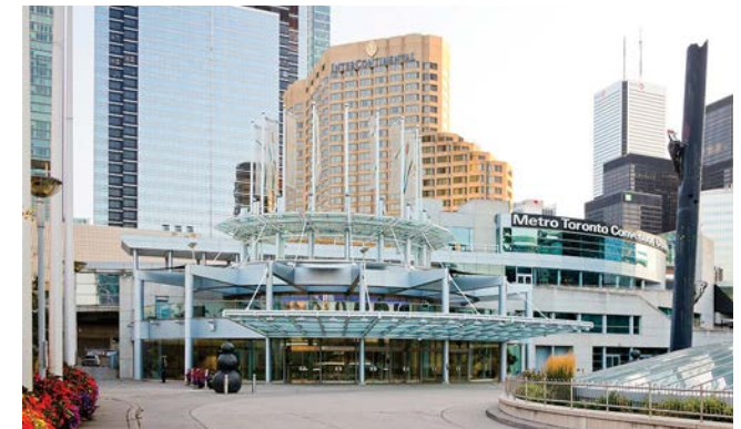
MTCC South Building
