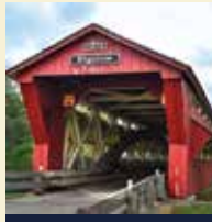
Length: 102 feet Year: 1873 Builder: Partridge Spans: Little Darby Creek Historical Marker
