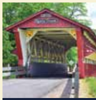
Length: 64 feet Year: 1883 Builder: Partridge Spans: Spain Creek Historical Marker
