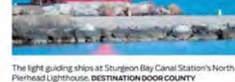
The light guiding ships at Sturgeon Bay Canal Station's north Peninsula Lighthouse. DESTINATION DOOR COUNTY
