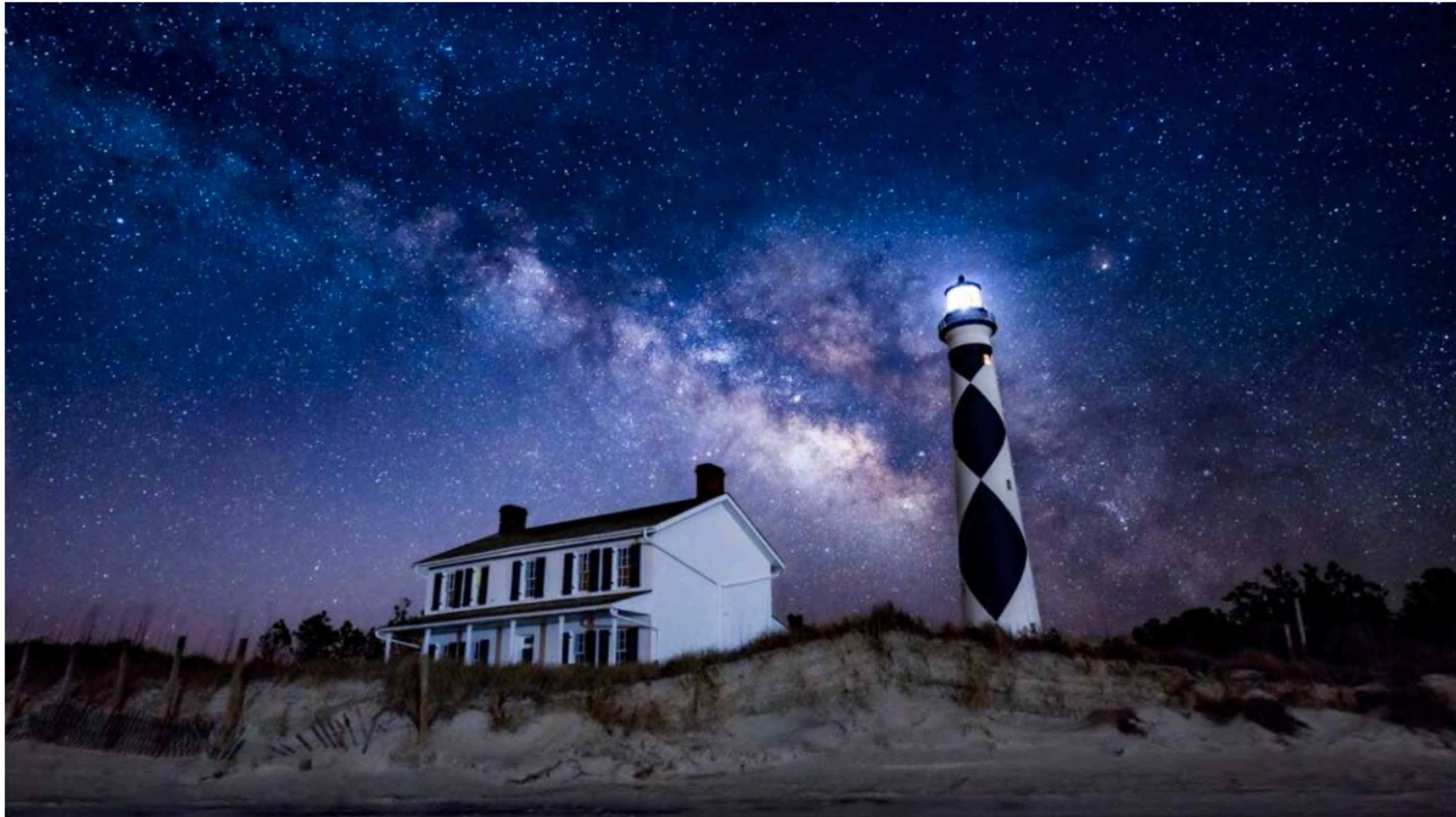
A dark, clear night displays the Milky Way over the Cape Lookout Lighthouse and the keeper's quarters in this undated photo. Cape Lookout National Seashore has been named an International Dark Sky Park. (Alex Gu photo)
