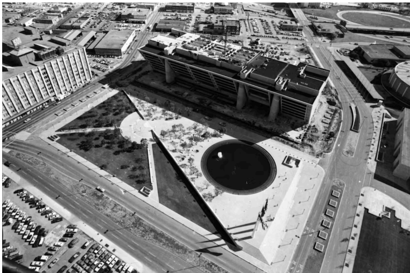
Aerial view of I. M. Pei's City Hall and plaza under construction in 1976.
