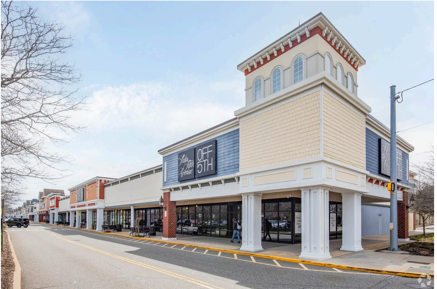
This Saks Off 5th store in Riverhead, New York, is among the nearly 60 slated to close. (CoStar)
