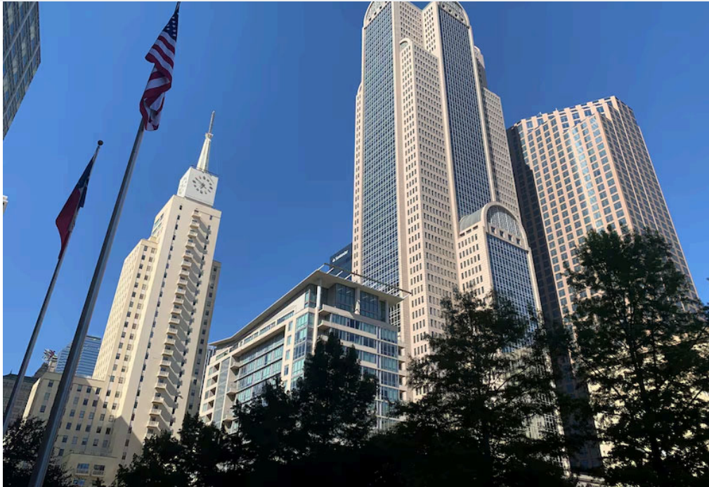
From left: the Mercantile Building, which is terminating all of its leases due to a leak and noxious odor; the Comerica tower, whose namesake tenants are eyeing an Uptown move; and 1700 Pacific, which is a shell of its former self.
